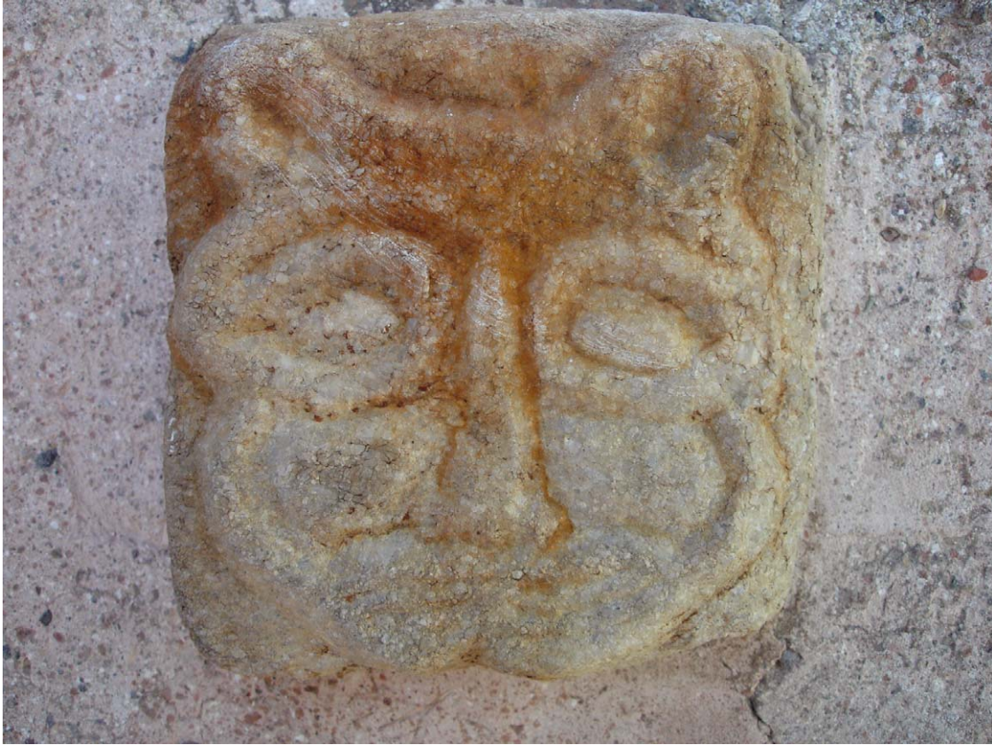
19 Vatopedi monastery; bell-tower; outer northern façade; marble brick
