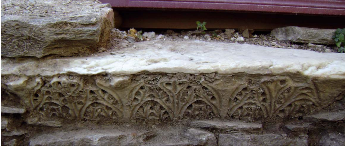
17 Skete of St Demetrios; kyriakon; part of a cornice impacted in the stone-built krepis
