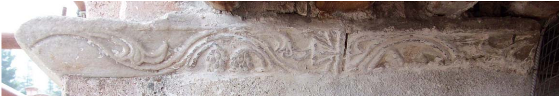
10 Vatopedi monastery; bell-tower; eastern wall-opening; part of a cornice on door frame with unfinished sculpted decoration, impacted in the southern arch
