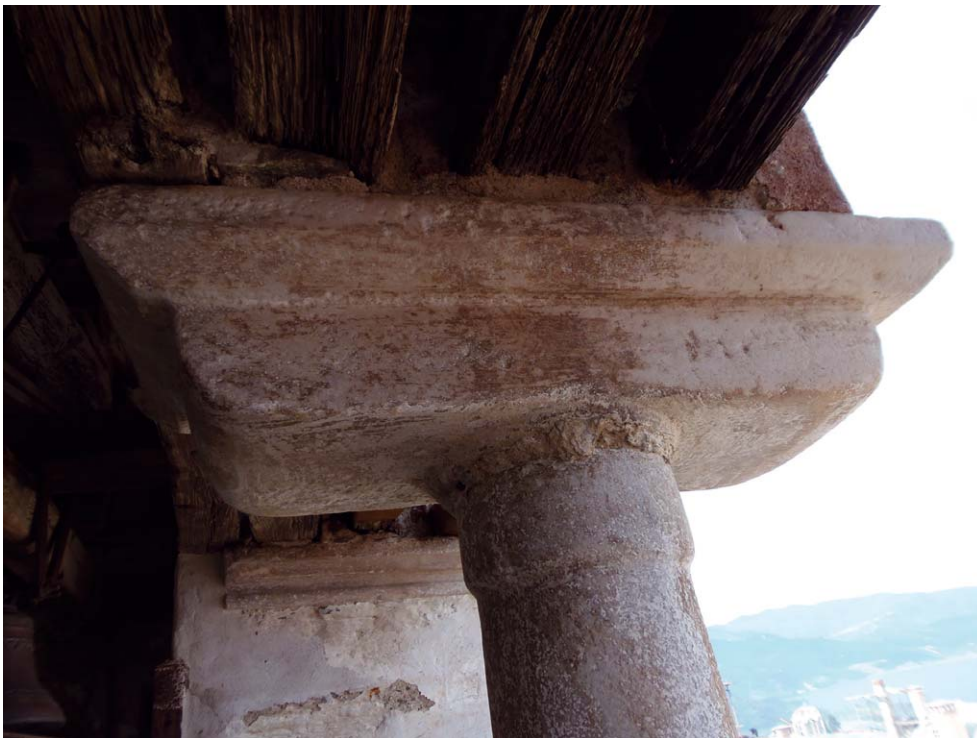
7 Vatopedi monastery; bell-tower; capital with inherent impost of the column (wall-opening, northern façade)
