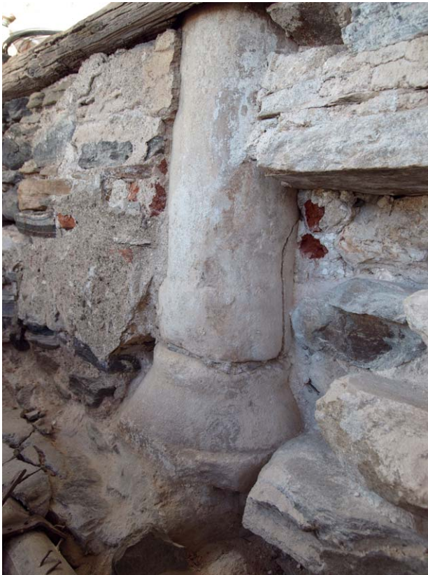
6 Vatopedi monastery; bell-tower; the lower part of the column with the base in the wall-opening of the northern façade
