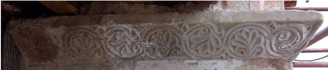
11 Vatopedi monastery; bell-tower; eastern wall-opening; part of a cornice impacted in the northern arch
